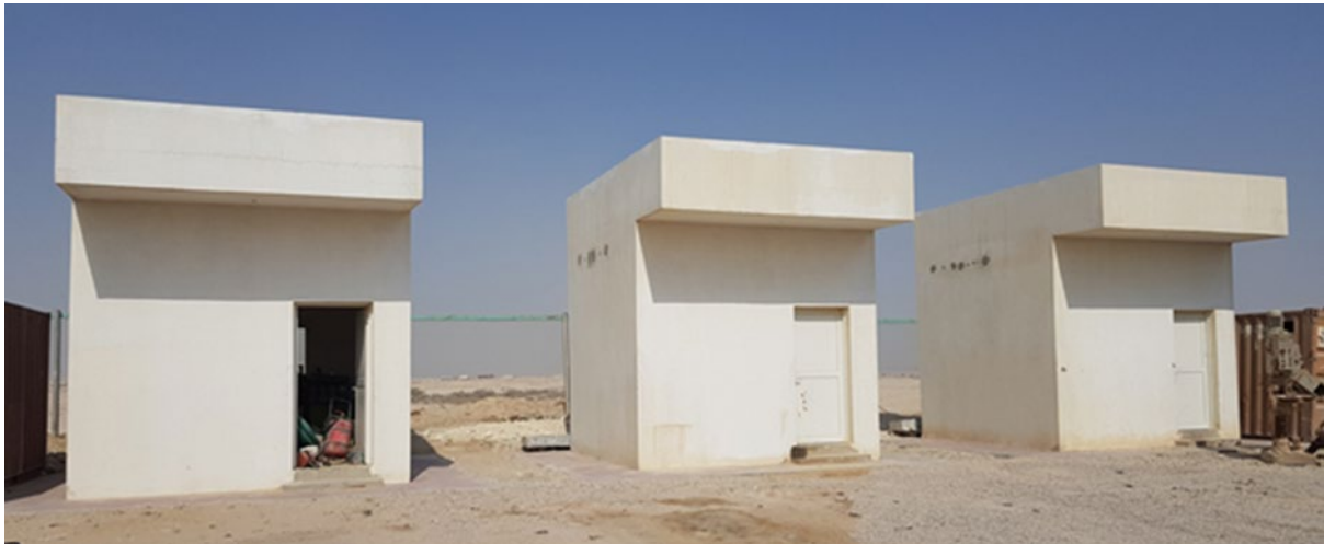
Figure 3. Trial buildings, 4 years after construction: control (100% gabbro) on left; 50% Wadi gravel in centre; 100% Wadi gravel on right
